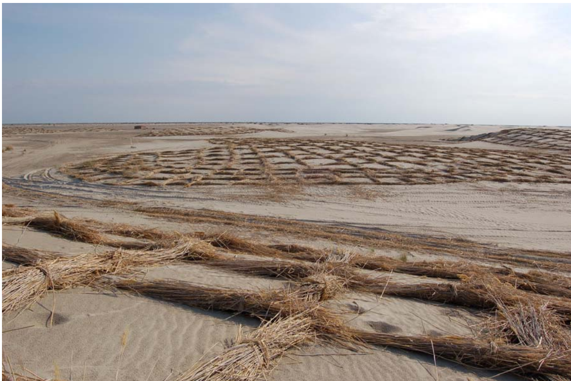
Fig. 11: Mechanical fixation of moving sand with reed cane
