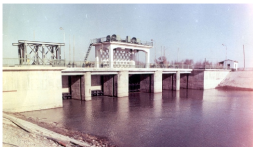
Headwork structure of Turanga Saka Canal
