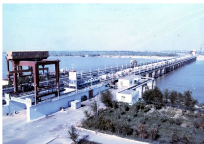
Barrages of Takhiatash hydrounit (Nizhnedarya Division)
