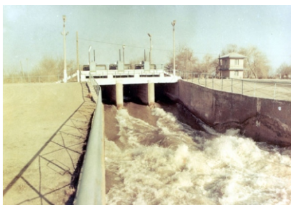
Recharge structure within 42 km of Shavat branch canal
