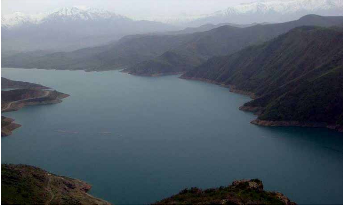
HEPS dam forms the Gissarak reservoir for seasonal flow regulation with the total volume of 170 Mm 3 and available capacity of 162 Mm 3
