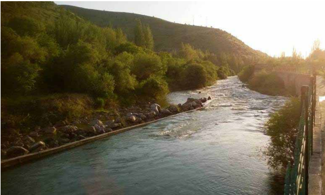
Diversion canal in tail race of the Gissarak hydroscheme
