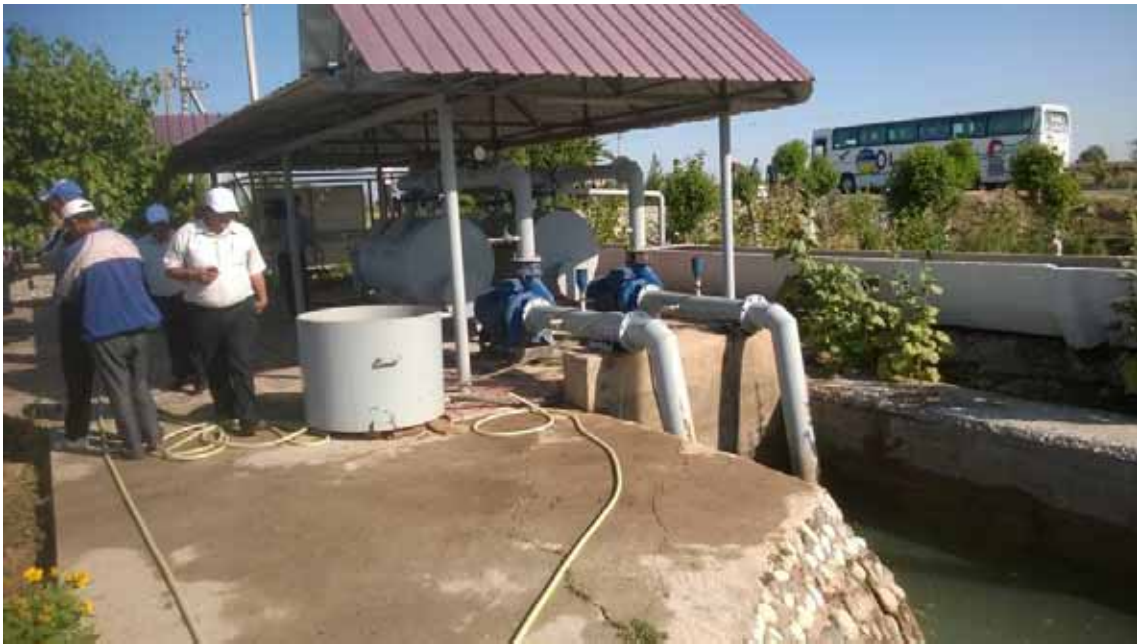
Pumping and filtering equipment for drip irrigation system
