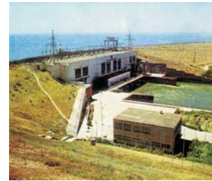
• Hydro structure on Chardara reservoir
