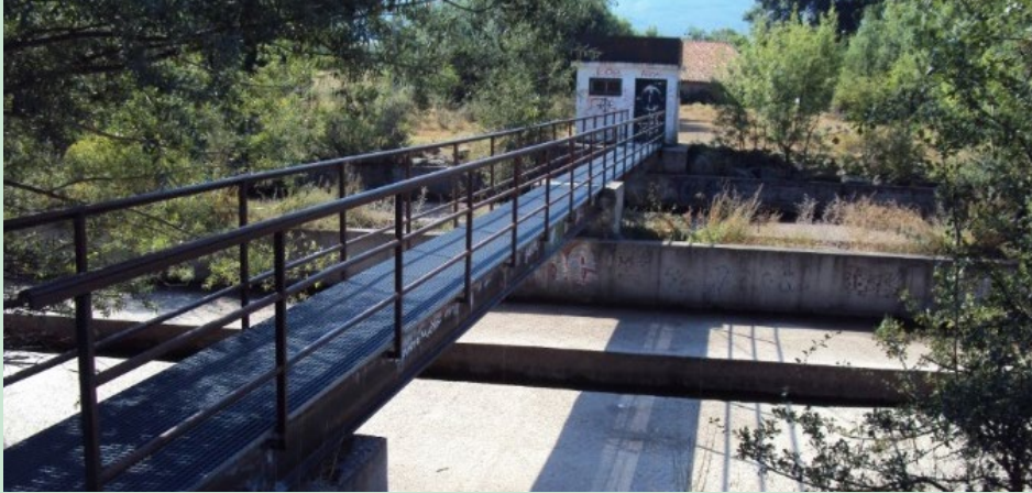
Abandoned gauge station on the river Lozoya
