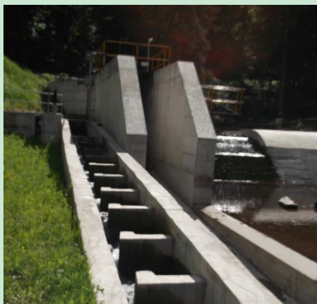
1 - Water intake and fish pass—Micro Hydropower Plant Budac I, Bistrita-Nasaud County 2 - Wastewater Treatment Plant – Carei Town, Satu Mare County
