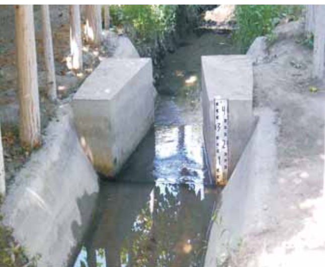
Hydrometric post with a water metering device similar to “SANIIRI” flumes.
