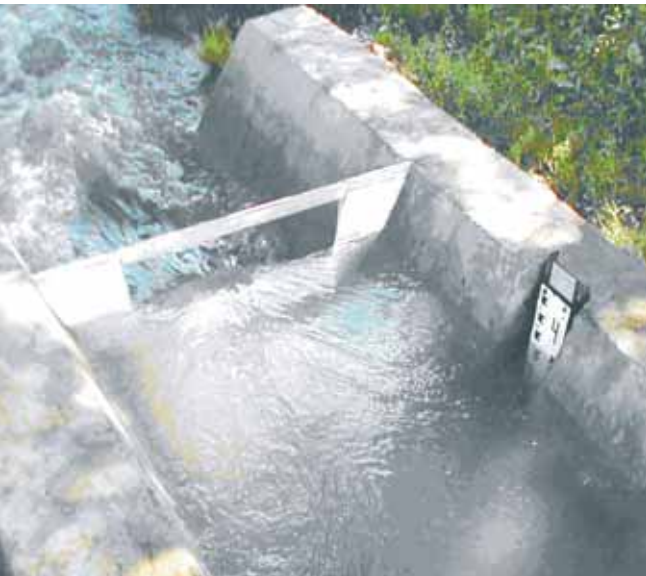
Association canals are equipped with standard water metering devices similar to “Chipoletti” weirs, “SANIIRI” flumes, etc.
