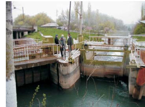
Structure on PK-70 of Aravan-Akbara Canal, Osh province
