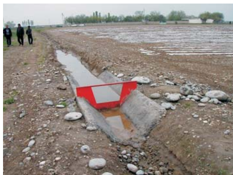
Water metering device in the field, farm "Navoi" in Fergana province
