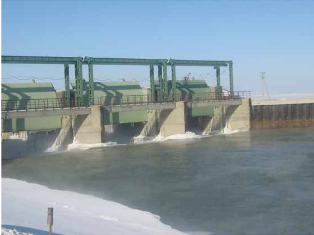
Figure 7 – Aklak water-retaining structure (2009)
