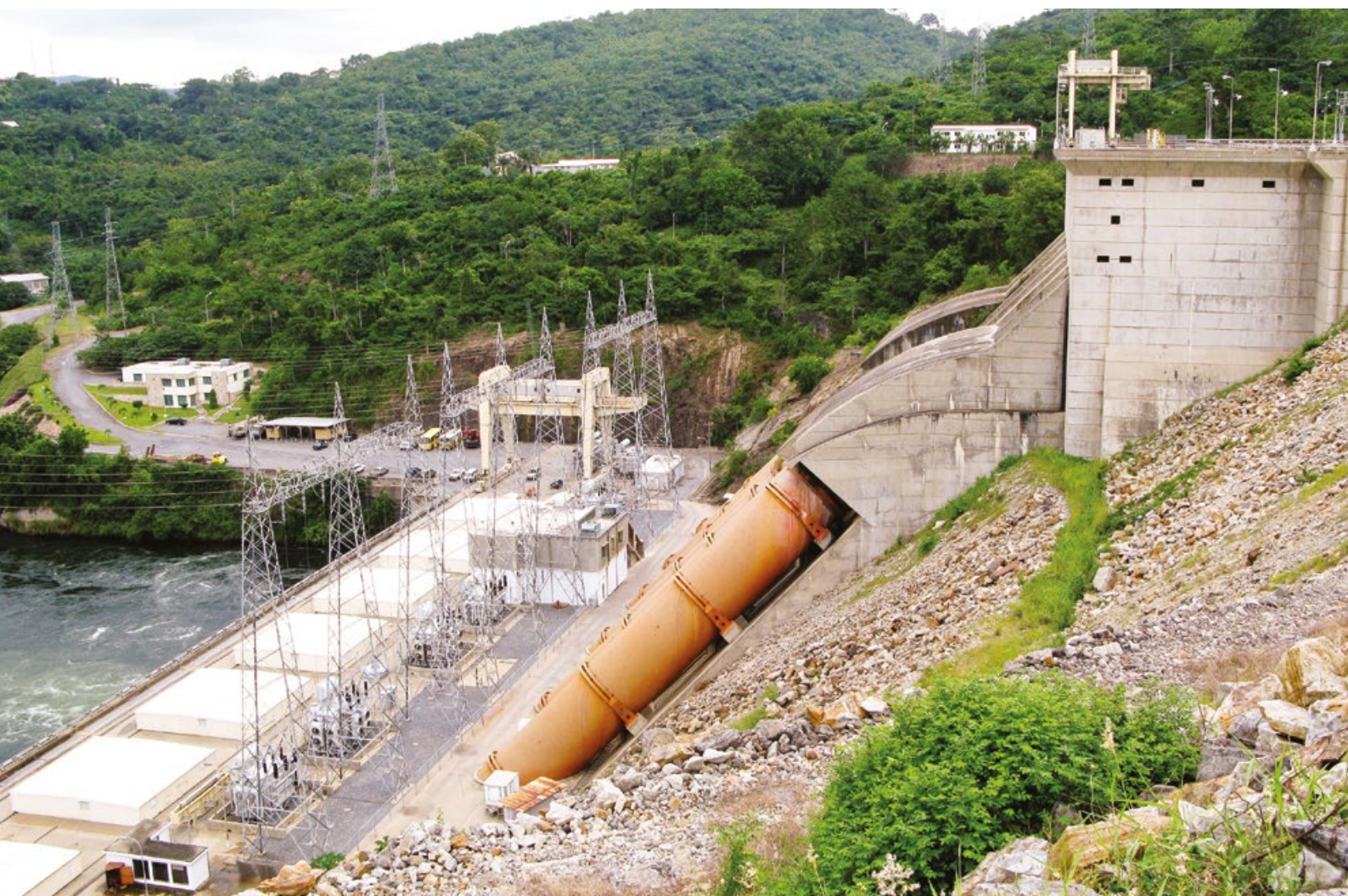
Hydropower plant in Ghana
