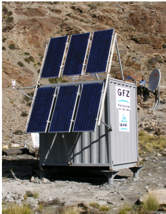
Automated monitoring stations deliver reliable weather and flow data from the high mountains in real time.
