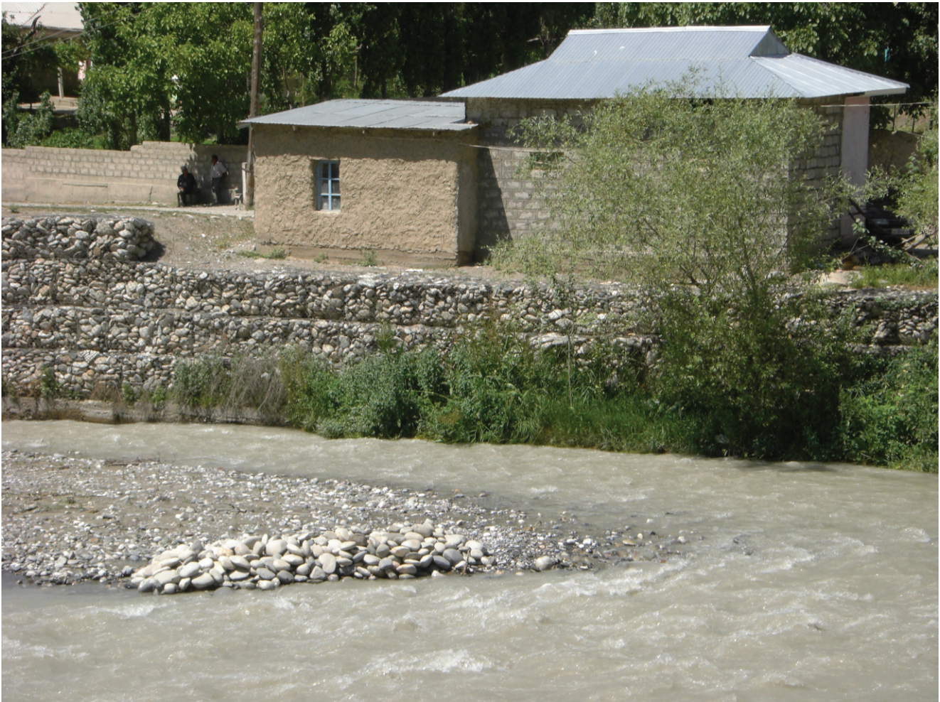
FIGURE 7 In the upper part of the watershed, stonewalls have been constructed to protect homes close to the riverbank from flash floods. Khozho-Bakyrghan WUA, Kyrgyzstan. (Photo by Dominic Stucker, 2011)
